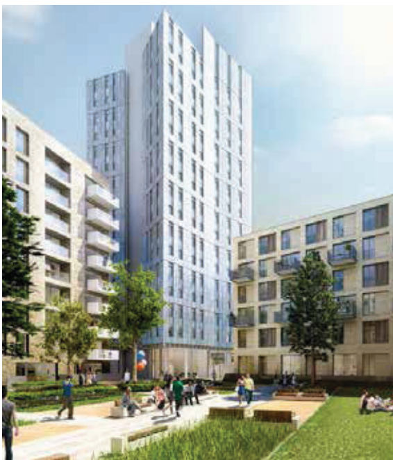
Figure 3.62 Taller building on the Westfield site
