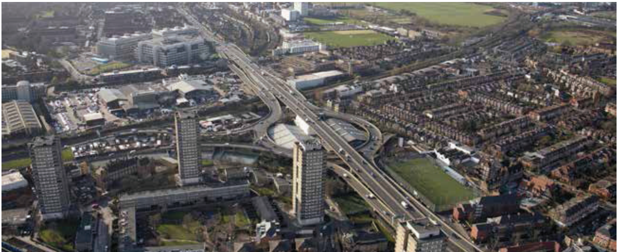
Figure 3.57 Aerial view of the Westway - existing
