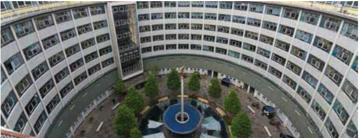
Figure 3.41: BBC TV Centre, Inner courtyard
