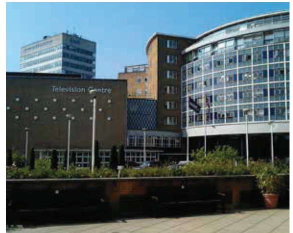
Figure 3.40: BBC TV Centre, Studio 1 and main entrance
