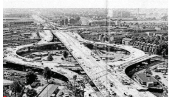
① Construction of the Westway (1960s)
