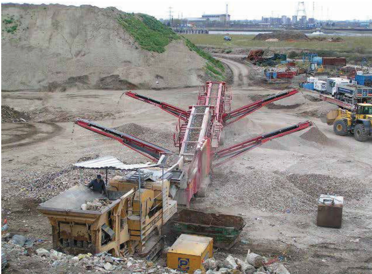
Figure 6.4: An example of on-site sorting and reuse of construction materials. (Source: Environment Agency 2012)
