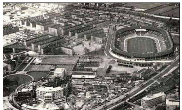
④ BBC TV Centre under construction
