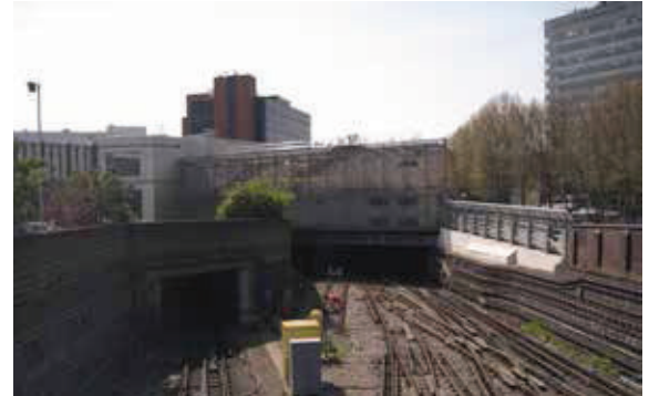
② Central Line cutting
