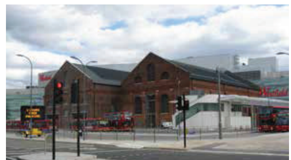
(C) DIMCO building
