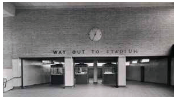
③ White City LUL Station, Central Line
