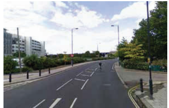
Figure 3.45: South Africa Road
